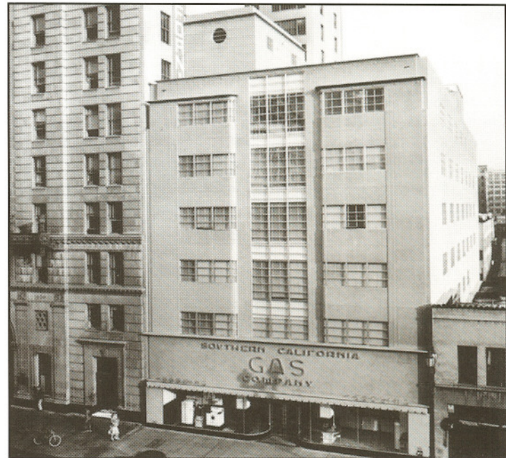
The First United Methodist Church sold the land at 8th and Hope to the Southern California Gas Co. in 1982, giving it enough money to fund programs and purchase the site at Olympic Boulevard and Flower Street where it wants to build a mixed-use project.
